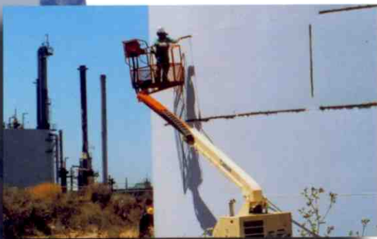
Bulk Storage Tank Demolition
