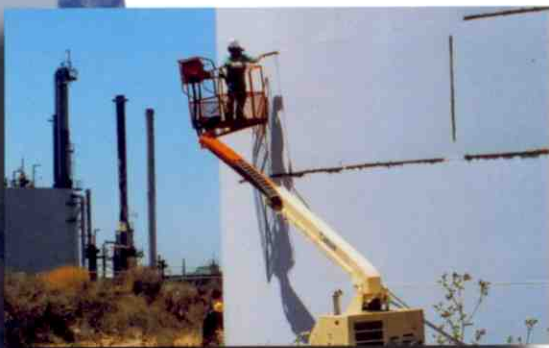
Bulk Storage Tank Demolition
